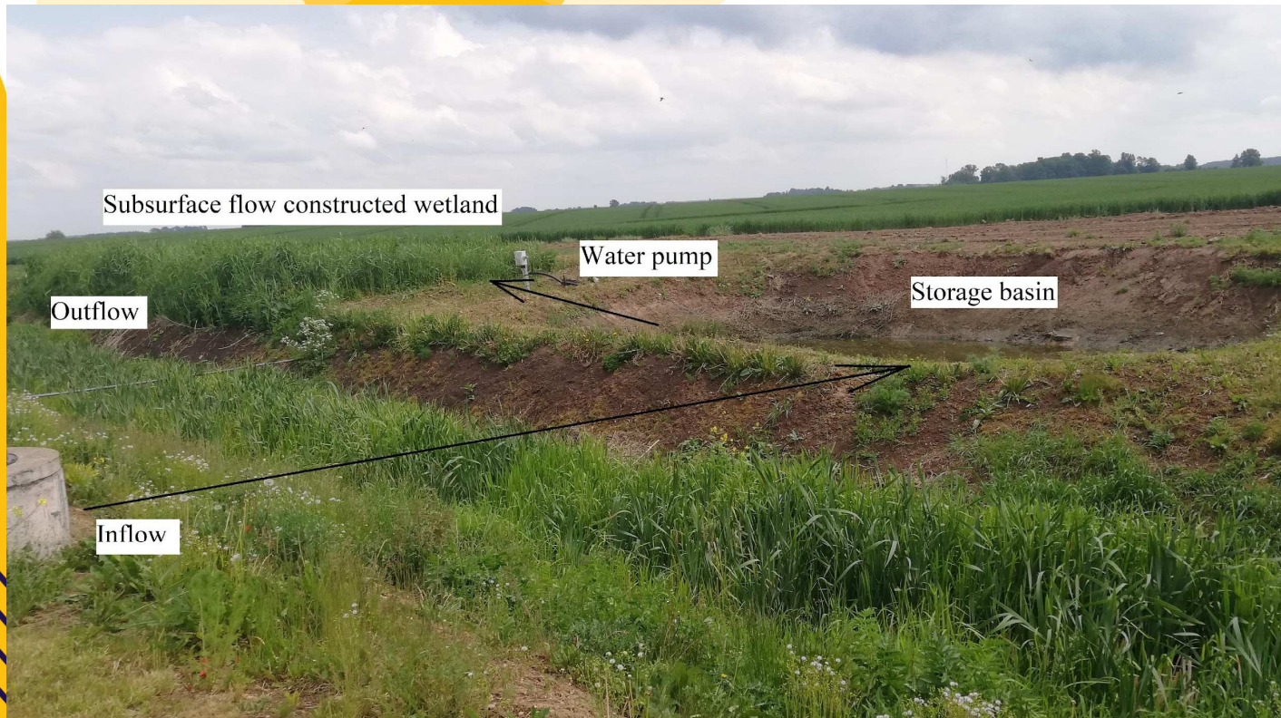
A storm water treatment system with horizontal subsurface slow constructed wetland at the Mezaciruli farm.
