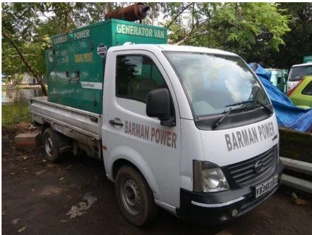
2.4.att. Elektroģenerators auto kravas kastē ( https://www.indiamart.com/proddetail/truck-mounted-silent-generator-19045337533.html )
